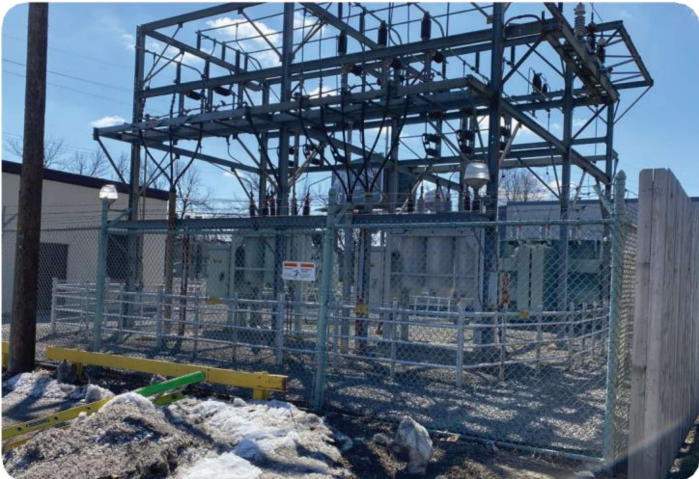
Existing metal support structure to be removed and replaced with modern, lower profile equipment.
