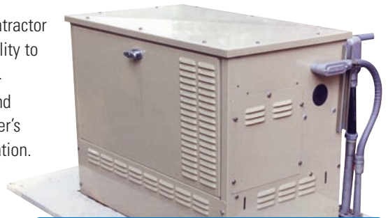
Typical stationary natural-gas fired generator
