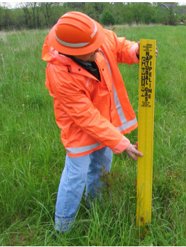
Line markers, such as the one above, indicate a buried natural gas pipeline's general location.
