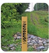
Since natural gas pipelines are underground, line markers are sometimes used to indicate their approximate location. The markers display the material transported and the pipeline operator's name and phone number. Markers only indicate a pipeline's general location and cannot be relied upon to indicate the exact position. Because many lines
