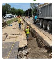
We have completed replacing and upgrading approximately one mile of underground gas main along South Winton Road in Brighton.
