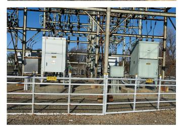
Of the two current control houses on the property, one will be demolished while the other will remain. A new GIS control house will be installed that will include state-of-the-art GIS Switch gear. Transformer banks #1 and #3 will be replaced and upgraded. Noise studies at the site have been within acceptable industry standards, and residential areas to the north are not impacted and benefit from a buffer of trees and natural vegetation boundaries.
