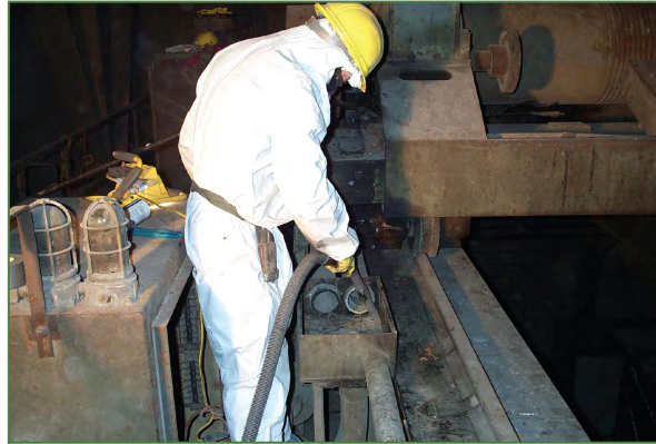
ASH REMOVAL WITH HEPA VAC SYSTEM
