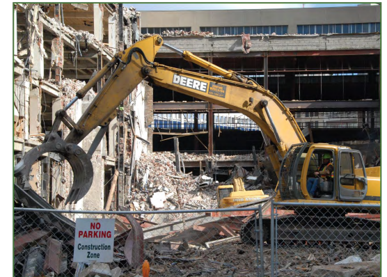
LARGE EXCAVATOR WITH GRAPPLER
