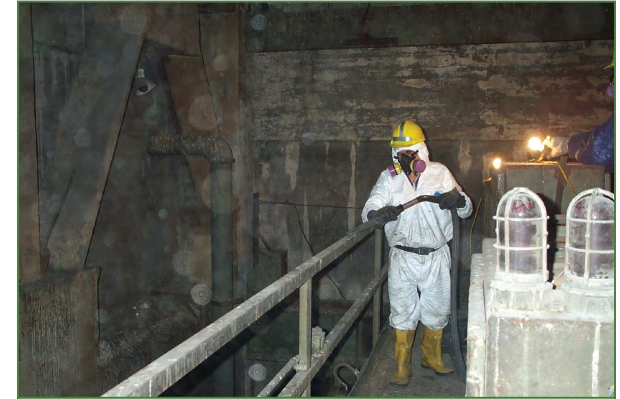
ASH REMOVAL WITH HEPA VAC SYSTEM
