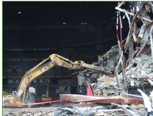
LARGE EXCAVATOR WITH SHEARS
