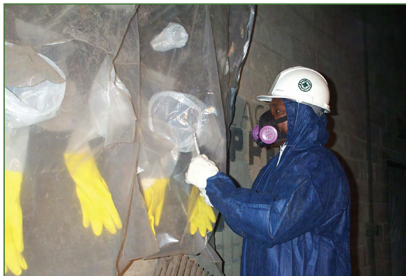
GLOVEBAG SYSTEM FOR PIPE TSI REMOVAL
