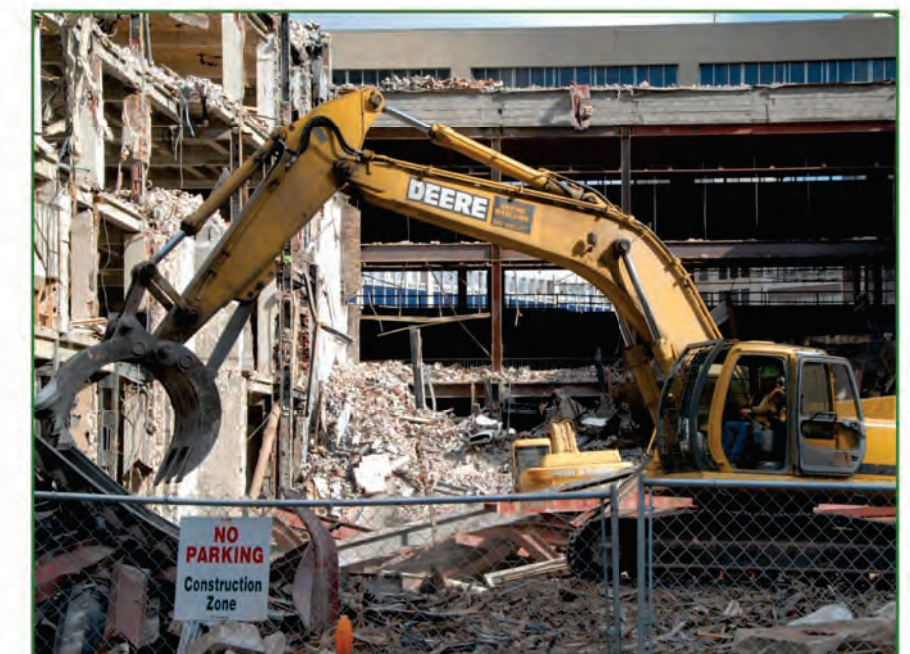
LARGE EXCAVATOR WITH GRAPPLER
