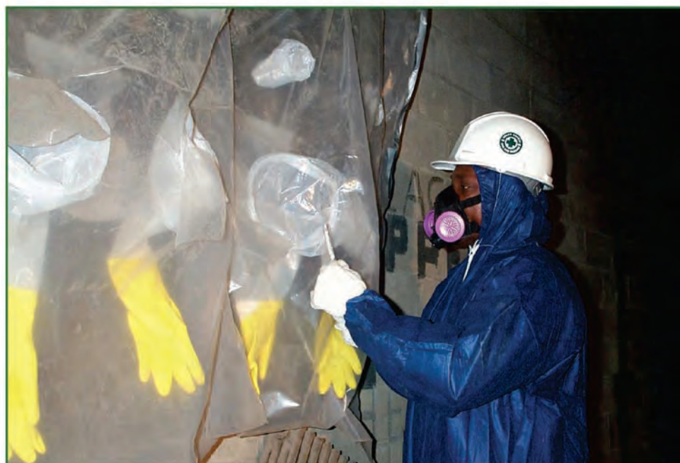
GLOVEBAG SYSTEM FOR PIPE TSI REMOVAL
