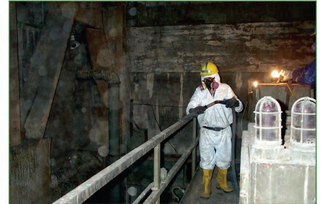
ASH REMOVAL WITH HEPA VAC SYSTEM
