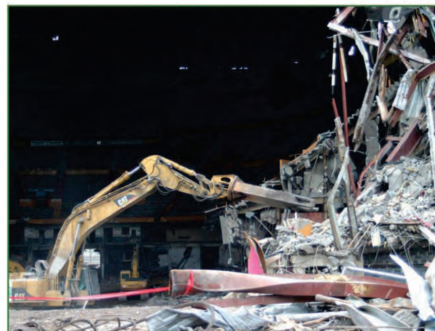
LARGE EXCAVATOR WITH SHEARS
