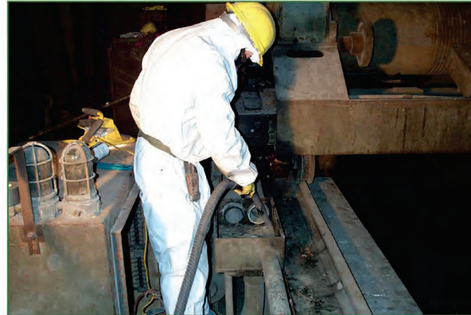
ASH REMOVAL WITH HEPA VAC SYSTEM
