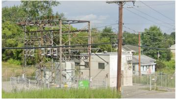
The facilities upgrade to Substation 156 will include an updated transformer, state-of-art gas insulated switchgear (GIS) technology, an On-Load Changer (OLTC) transformer bank, and the conversion of three existing distribution lines to more robust capabilities. Additionally, a new Control House and corresponding new perimeter fencing will be built at a different location within the property. Contingency lighting will also be installed to allow for any urgent afterhours work.
